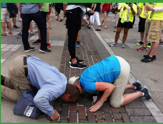
See, there's some grout missing..
